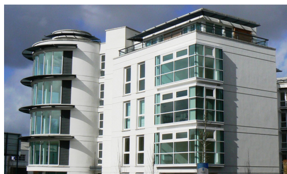
Apartments East Hill, London (UK)
