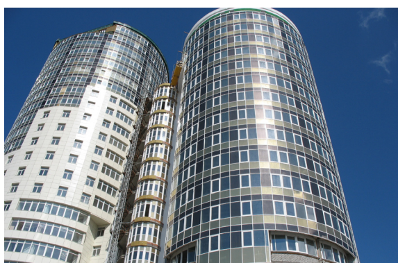
Apartments, Jekatarinburg (Russia)
